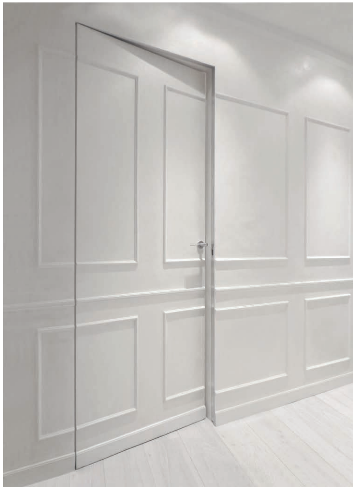
Hidden door in classical interior
